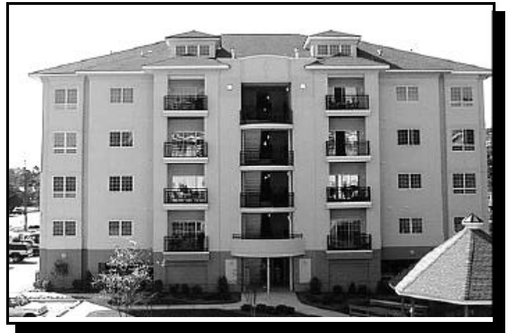
Open stairwells and stair landings are easily visible. Balconies and windows provide good surveillance.
